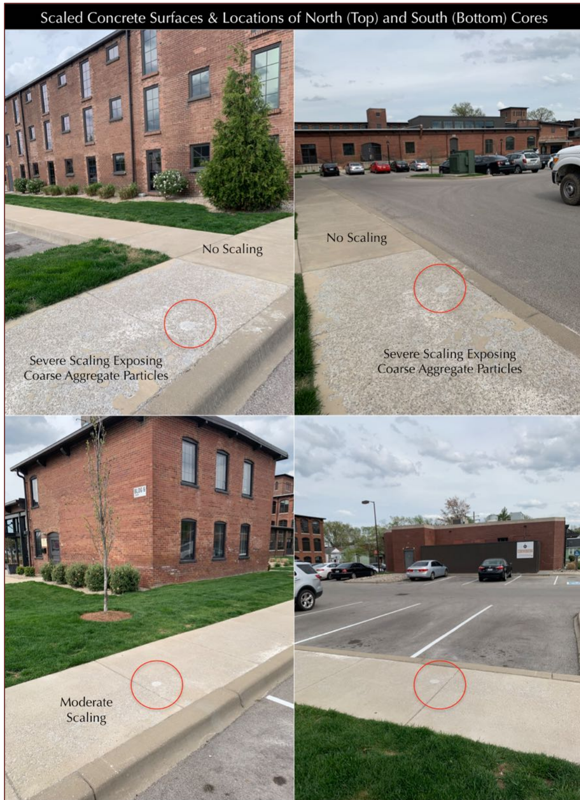
Figure 1: Field photographs of concrete surface scaling at the locations of two cores (circled) marked as 'north' (top photo) and 'south' (bottom photo). Notice: (a) severe scaling of concrete surface and exposures of coarse aggregate particles at scaled locations of 'north' core in the top photo, (b) relatively lesser degree of surface scaling but exposure of coarse aggregate particles at the scaled location of 'south' core (bottom photo), and, (c) noticeably sound concrete slabs adjacent to the scaled ones of this investigation separated by construction joints.
