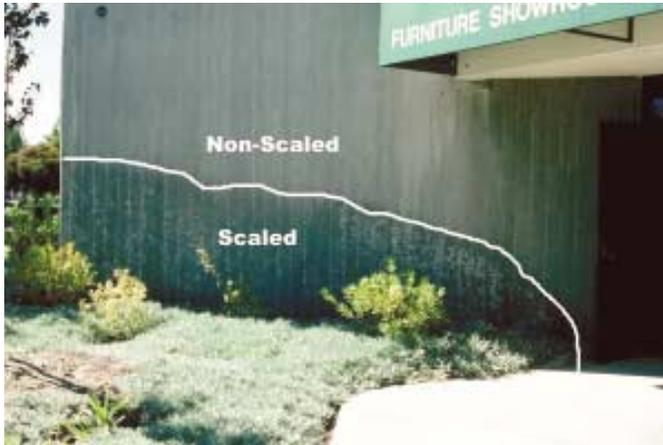
Fig. 10: Surface scaling due to cyclic conversion of laumontite to leonhardite at a location exposed to periodic water spray from sprinklers
