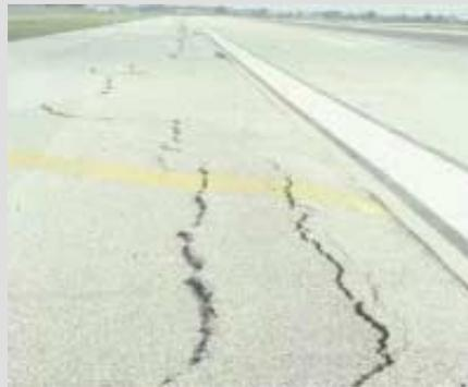
Fig. 8: "Thrust faults" in an asphalt shoulder flanking a concrete pavement expanding laterally due to electric furnace slag aggregate that contained free lime and periclase in an econo-crete subbase (concrete lean in portland cement)
